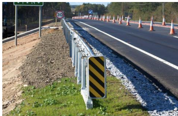
An example of an energy absorbent end terminal from the United Kingdom.
