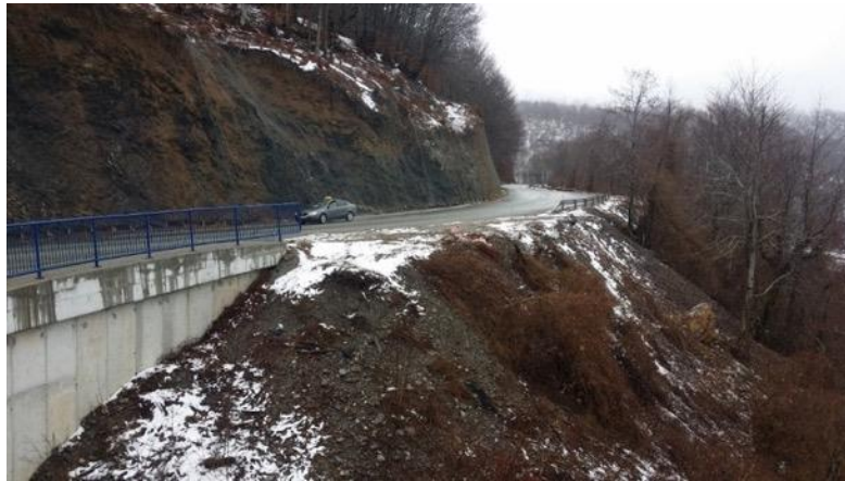
Example from Section One – gap in crash barrier between steel barrier and bridge parapet.
