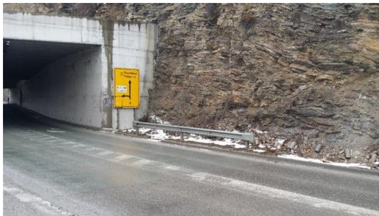
Existing underpass in Section Two – underpass headwall forms a roadside hazard and unsafe barrier terminal is also unsafe.
