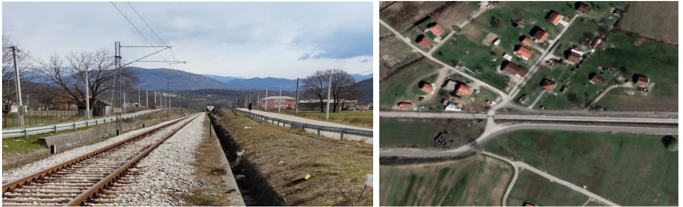
Figure 22. Level Crossing Šunjine
