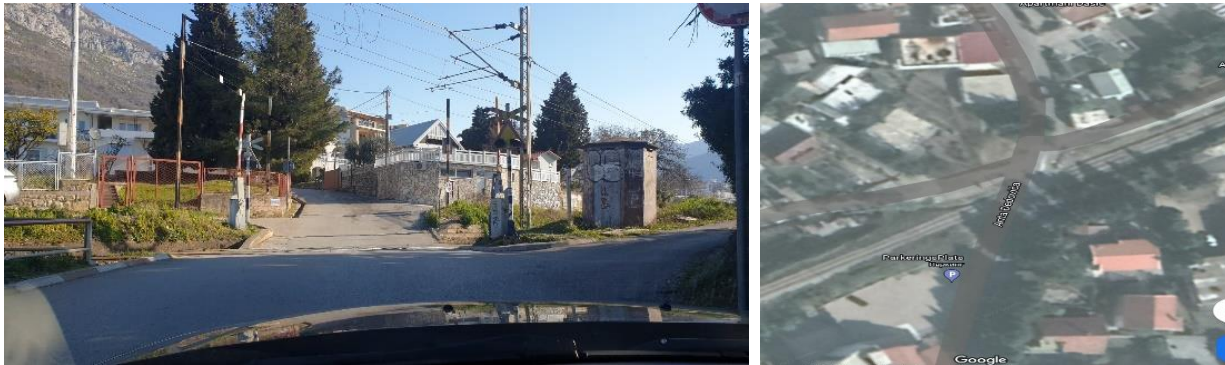
Figure 32. Level Crossing Žutokrlica
