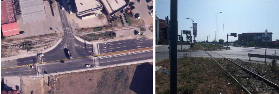
Figure 37. Level Crossing Peje 1
