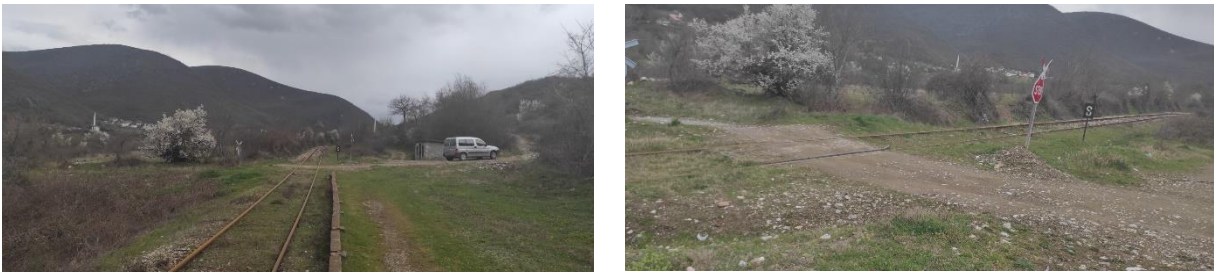
Figure 61. Orasje LC at km 022 + 207
