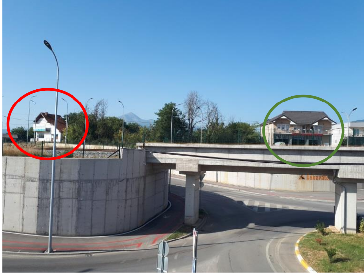
Figure 43. Level Crossing Varosh in 2021 (Underpass in Varosh)
