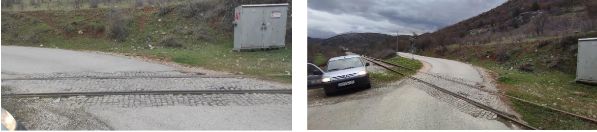
Figure 60. Orasje LC at km 020 + 590
