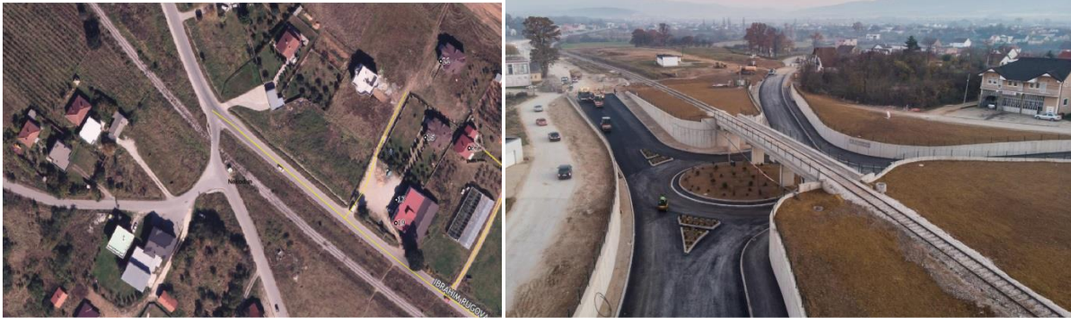
Figure 41. Construction phase of the underpass in Varosh, Ferizaj
