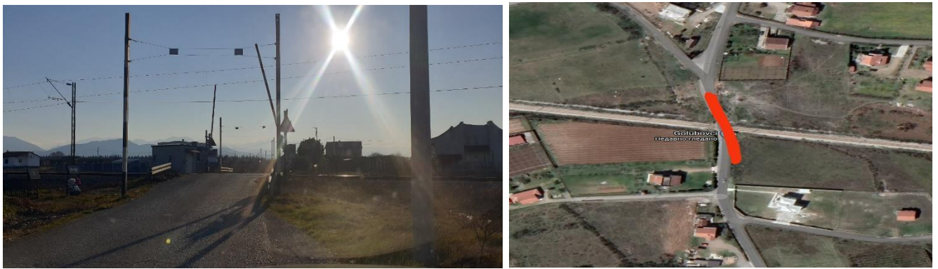
Figure 27. Level Crossing Mahala
