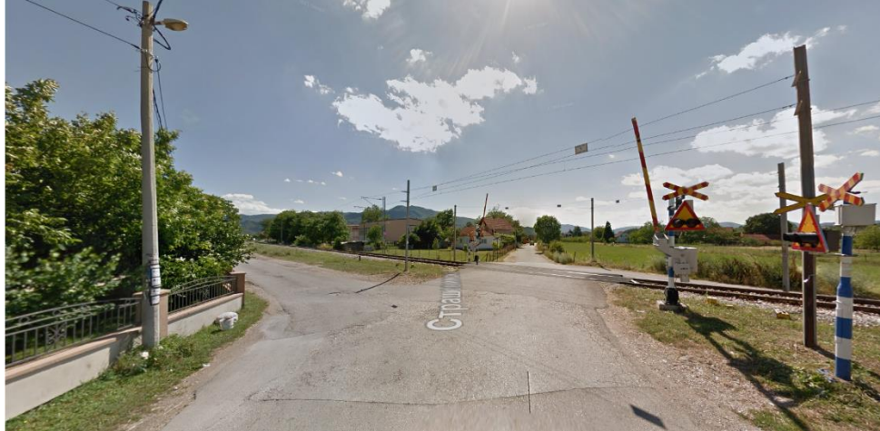
Figure 14. Level crossing "Klicevo"
