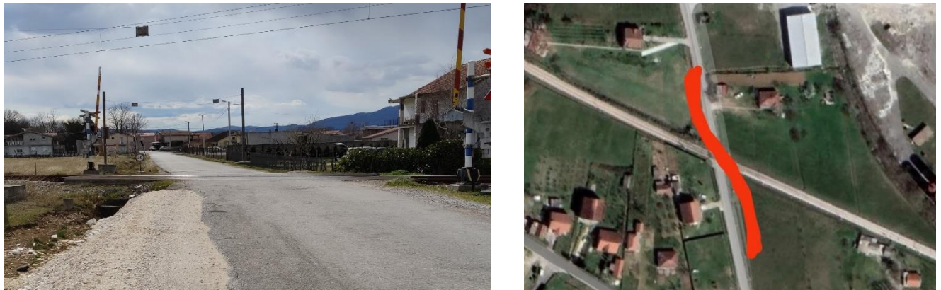
Figure 21. Level Crossing Burum
