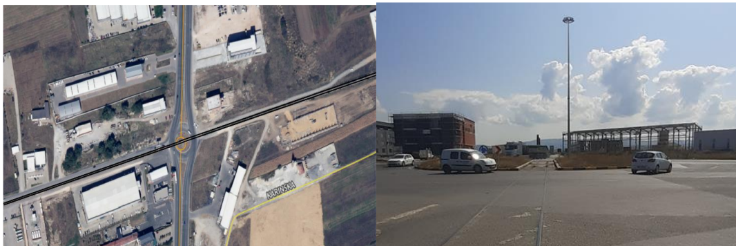
Figure 40. Level Crossing Gracanica
