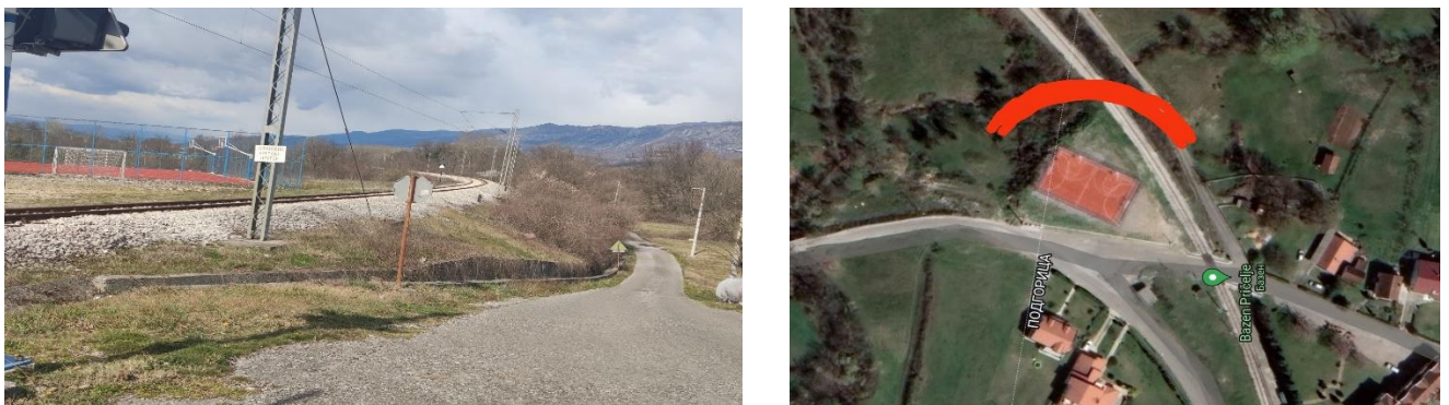
Figure 23. Level Crossing Pričelje
